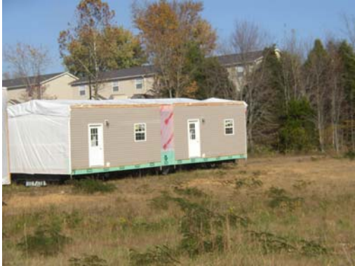
In preparation for setup, hinged roofs are raised.
