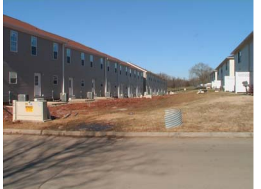
Air units are installed after all units are in place.
