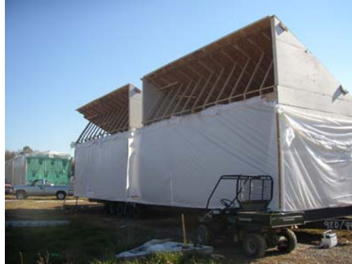
Bracing is installed in accordance with setup procedure.
