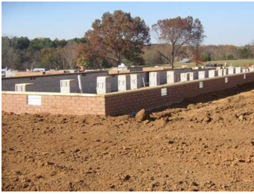
The foundation is prepared for the units prior to delivery.
