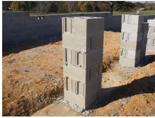
Perimeter & center piers are built same as in onsite construction.
