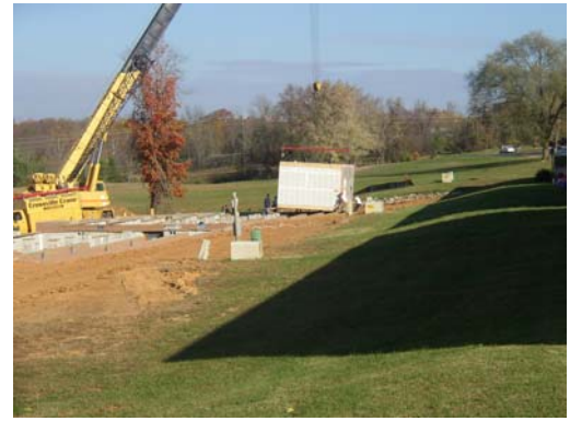
The rigging is then removed in preparation for the next lift.
