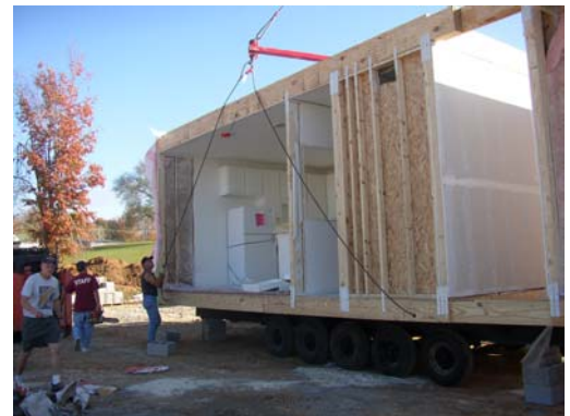
Rigging must be balanced before lifting the units.
