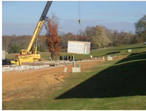
It is then positioned over the foundation and lowered.
