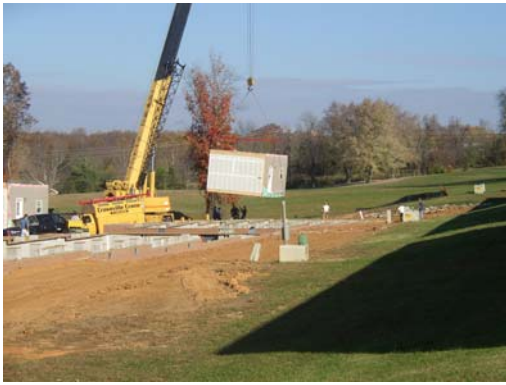
The unit is carefully lifted and moved into position.
