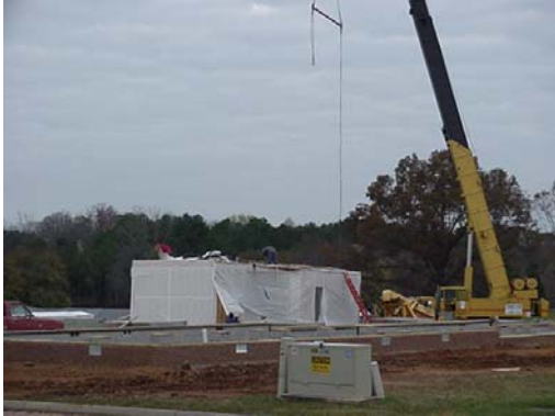
The first floor is set and positioned on the foundation.
