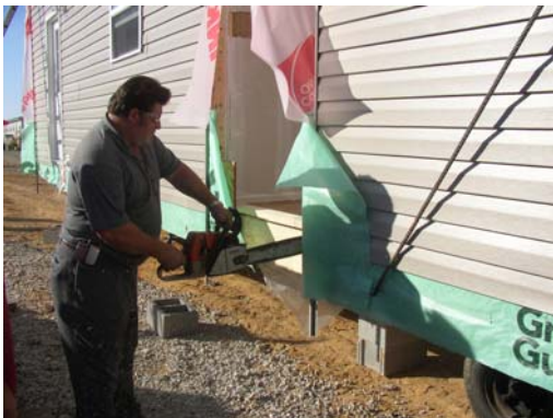
Units are separated in the field prior to installation.
