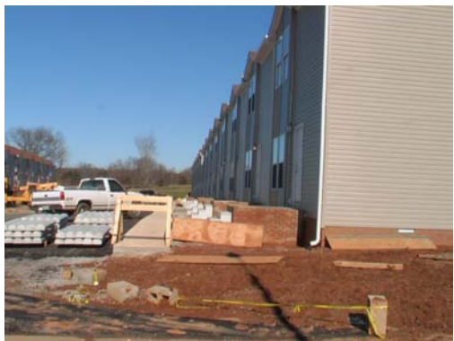
Building materials are cleared for landscaping and paving to begin.
