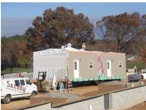
Exterior shipping material is removed before unit is lifted with crane.
