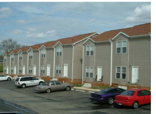
Final touches and inspections are made before occupancy of units.
